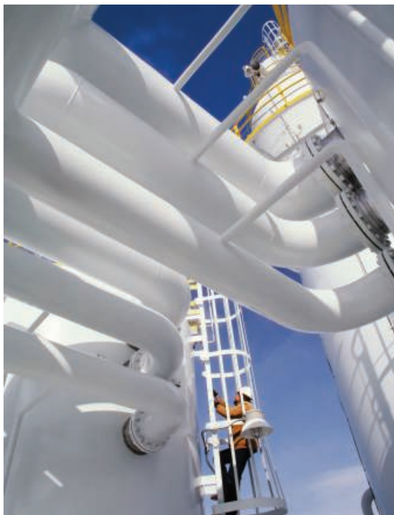
FIGURE 1. HAZOP studies are useful tools in reducing process risk, and they provide safeguards against hazardous scenarios for the personnel who must maintain and operate the plant
