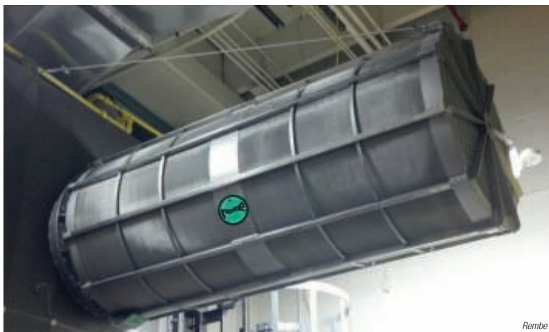
FIGURE 5. Rembe's Q-Rohr-3-6T/6T-AL is ATEX-approved for indoor flameless explosion venting of dusts, gases, hybrid mixtures and metal dusts
