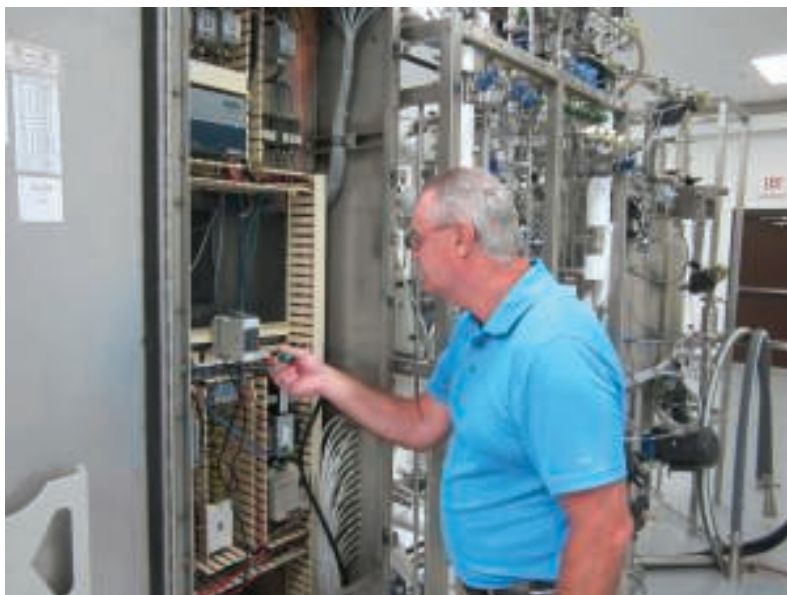
FIGURE 3. The ability to test in-situ validates the functionality of the safety switch while reducing maintenance and downtime
