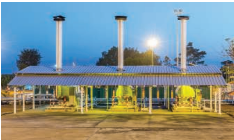
FIGURE 3. It is crucial that a HAZOP be explicitly targeted for the specific process in question, and not based on previous HAZOPs for similar processes, as process safety information and controls may have recently changed
